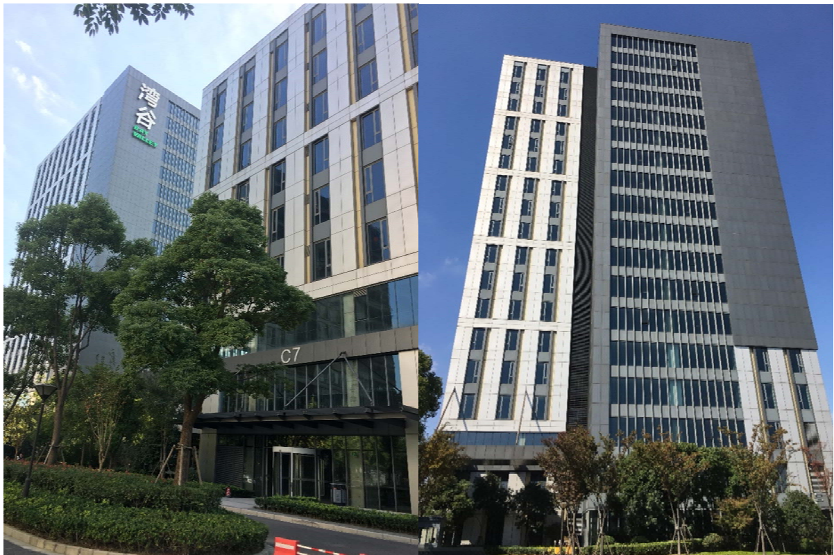
Metro's joint venture with Top Spring to acquire and operate three office buildings in Bay Valley, New Jiangwan City, Yangpu District, Shanghai
